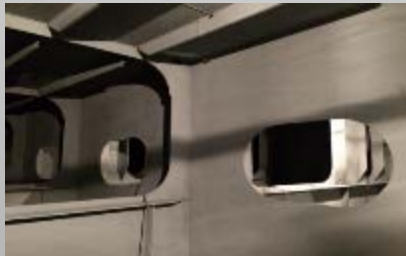
Methanol storage tank painted with zinc silicate
